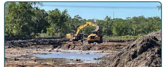
Construction activities south of 41st Avenue East
